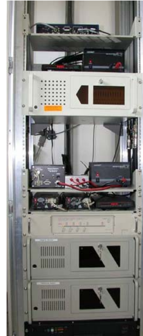
Figure 4 – ETRAN equipment rack at Eurofix station Sylt, Germany. From top to bottom are EGNOS receiver, modem & power supply, ETRAN PC, Eurofix receiver & power supply, 2 GPS receivers & modem, CPU switch, integrity monitor PC, Reference station PC, and a UPS at the bottom.
