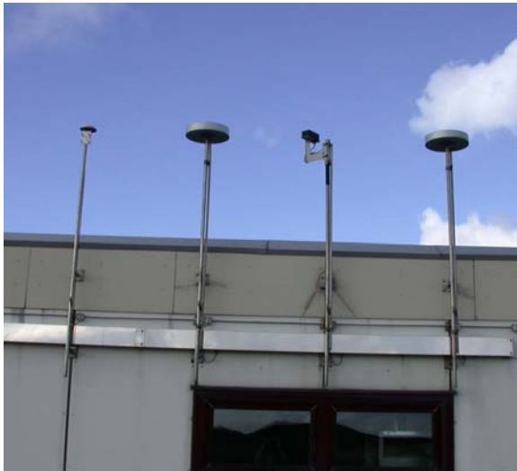
Figure 3 – ETRAN antenna setup. From left to right the antennae for the EGNOS SBAS, Eurofix integrity monitor, Eurofix data link monitor, and the Eurofix reference GPS receivers.
